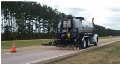
Asphalt rejuvenator is placed on U.S 25 near Jackson, Miss., using a BearCat 2,000-gallon distributor on an abraded surface.
